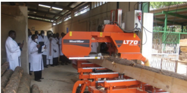
Board members visiting the main log conversion workshop newly installed Woodmizer machine has been installed
